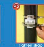
Position bracket at desired location on pole
